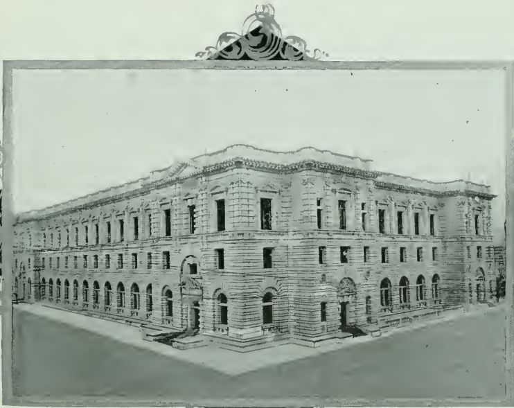
THE NEW POSTOFFICE. Cor. Mission and Seventh Streets.
